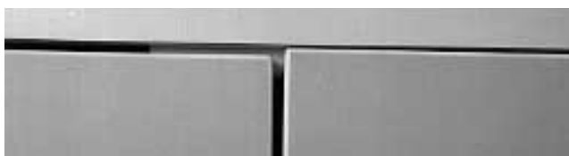
INCORRECT ALIGNMENT
