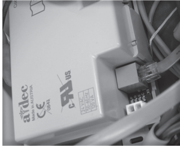
Figure 9. Plug in the Data Line
